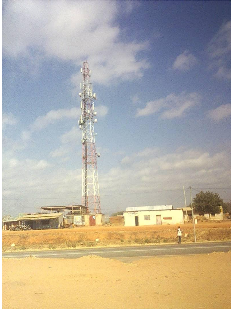
Figure 18: Communication Tower at Chemba Town, Chemba District
